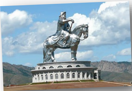
This model of Genghis Khan is currently the tallest equestrian statue in the world, standing 130 feet high (not including the museum building beneath it). Talk about being on your high horse!
